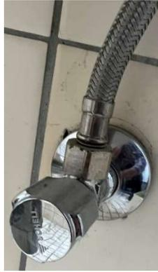
5. And screw the hose connection with the thread onto the wall connection and tighten it (be careful, "after tight it comes off" says the craftsman. Please make sure that there is a black rubber seal in the thread.
